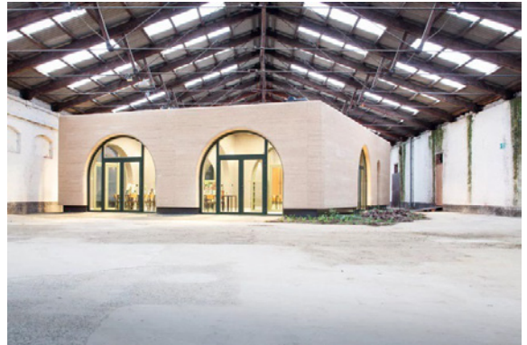
Figure 6. Fort V, Regional house of the Edeghehem commune, BC Architects. Regional House is a warehouse for children to learn about nature and ecology. The completed building reflects this educative and ecological approach through a radically sustainable and participatory architecture. Photo credit Thomas Noceto
