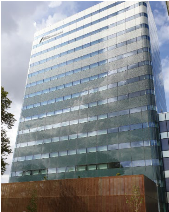
Interior roller blinds for solar control activated at Regionens Hus in Gothenburg. The last three windows on the right of the facade have no roller blinds as there is a fire escape staircase behind the glass. The bent corner glass is XTREME 70/33 just like the flat glass. The convex curvature reflects a larger part of the surroundings, which gives a glossy illusion of higher reflection.
