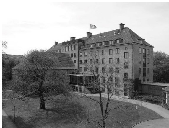
Figure 4. Denmark's Sankt Lukas Hospice, Denmark Source: www.fof.dk
