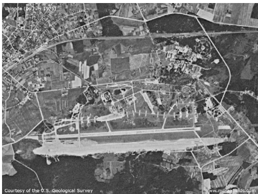
Figure 14. Enlargement - In the northeast, there is an anti-aircraft missile site (circular structure). Source: U.S. Geological Survey [map]
